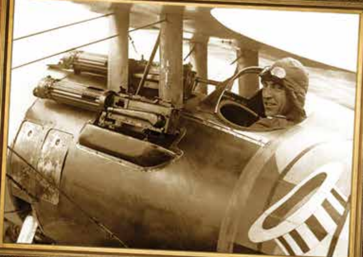
Leading American ace Capt. Eddie Rickenbacker in his Nieuport 28 with two Vickers. The narrow fuselage required offsetting the second gun.
