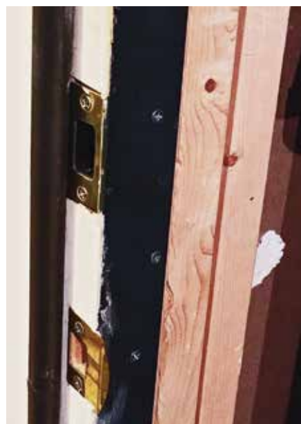
Simply drilling holes and screwing a piece of 1/8" steel bar behind the striker plate of your door frame adds a lot of strength to keep guns in and trouble out.
