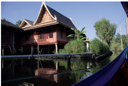
▲ Canalside home, Thonburi
