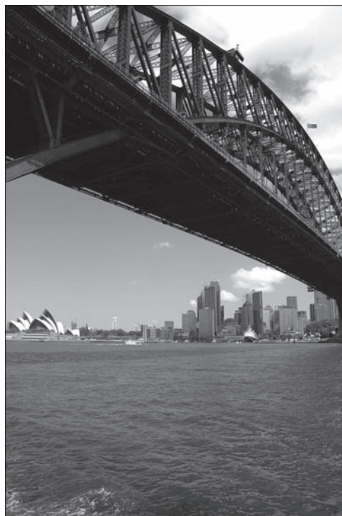
▲ Sydney Harbour Bridge
