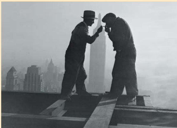
Rockefeller Center construction workers, 1932
